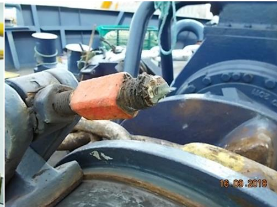
03b – Failed section of brake assembly
